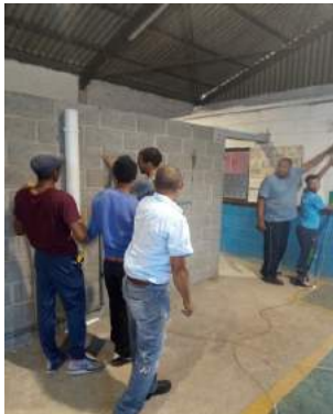
Neville de Villiers teaching plumbing students
