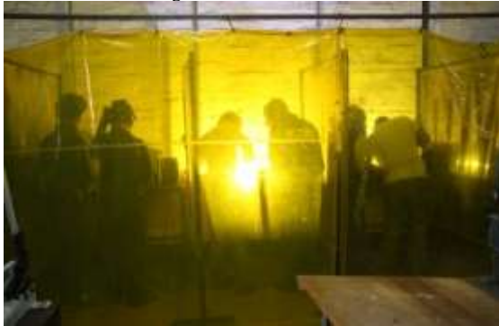
Pictures of the welding at RMI
