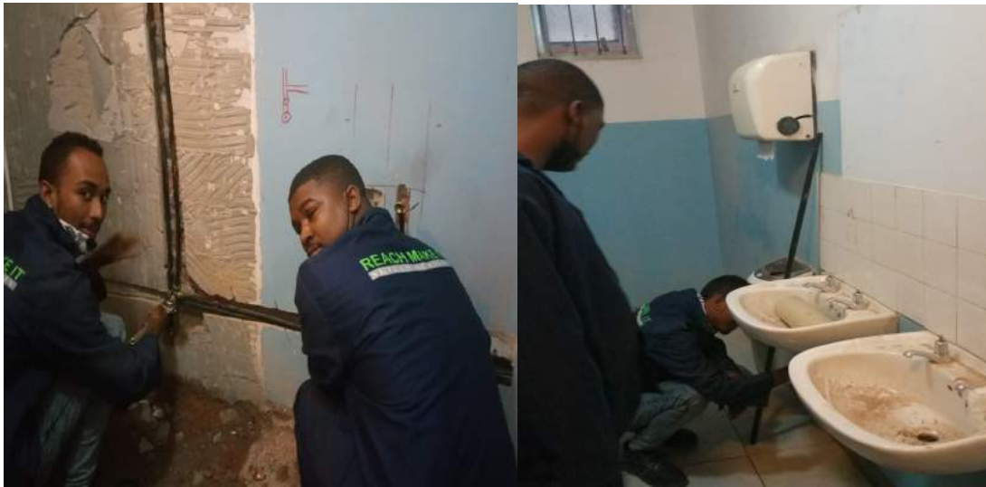
Here are the plumbing students of RMI busy doing the renovations at the STC Building
