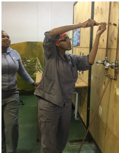
Students practising installation of sanitaryware and drainage system
