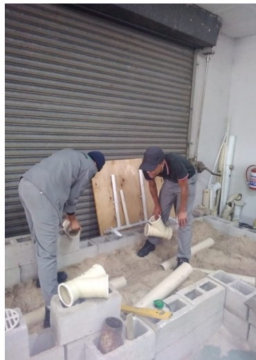
Students practising installation of sanitaryware and drainage system
